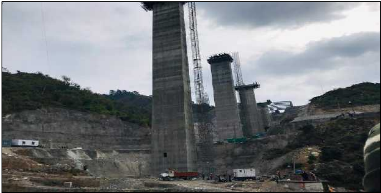
Reasi bridge piers
