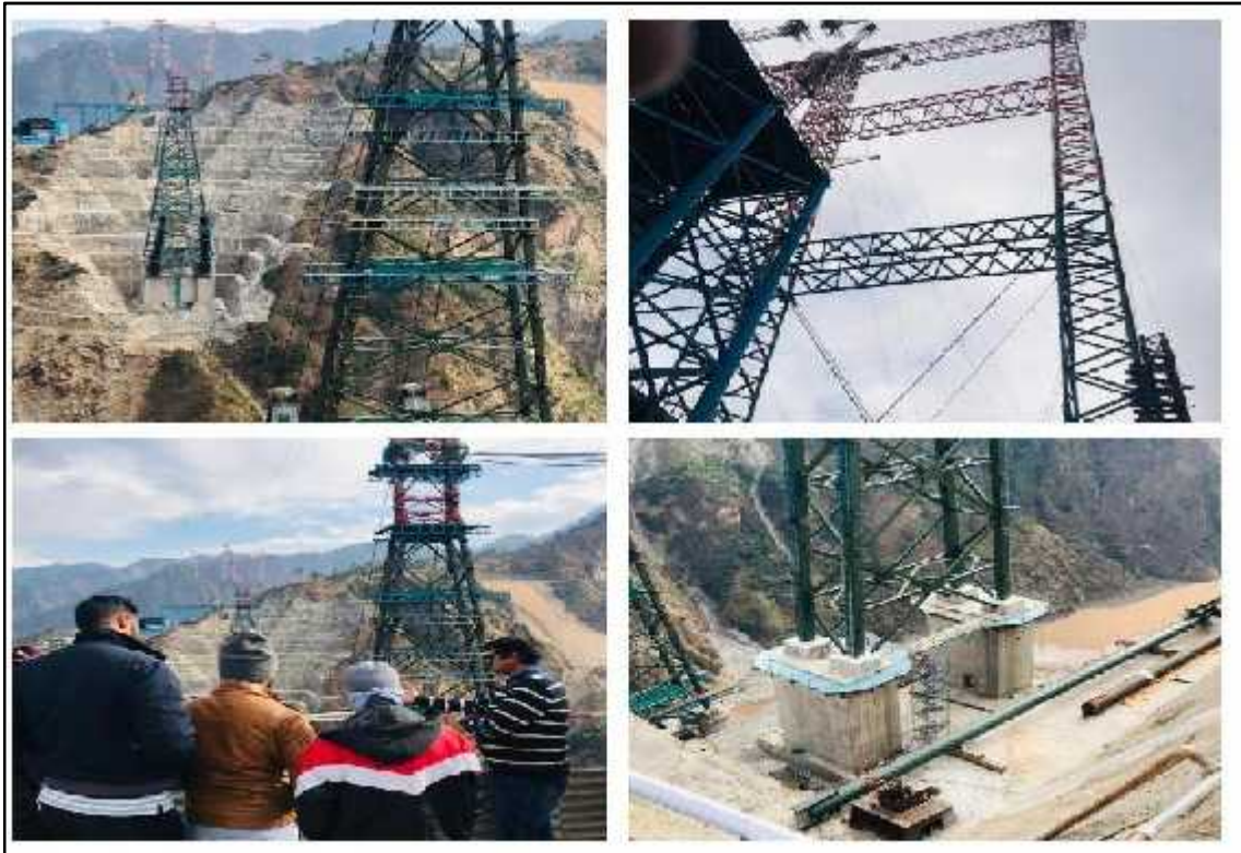
Chinab River Bridge construction
